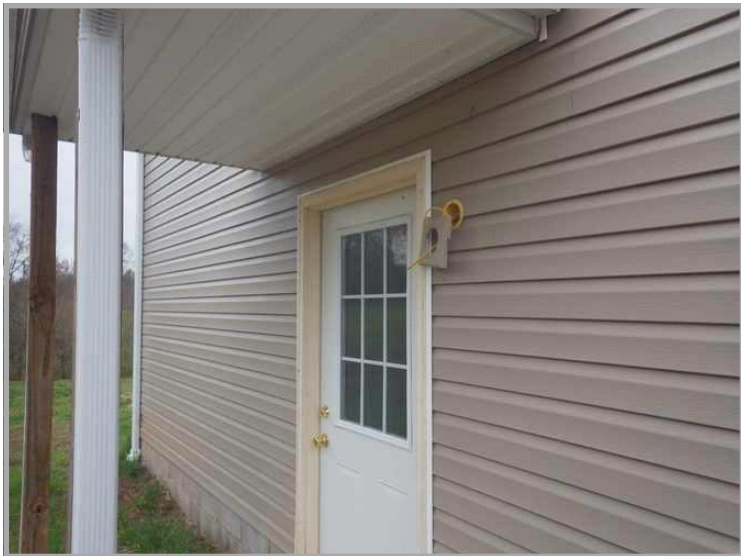
Incomplete Exterior Lighting
