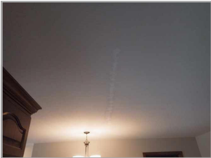
Ceiling Stain in Dining Area
