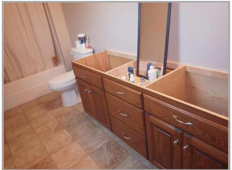
Owner's Suite Full Bathroom - Missing Sink Top & Fixtures
