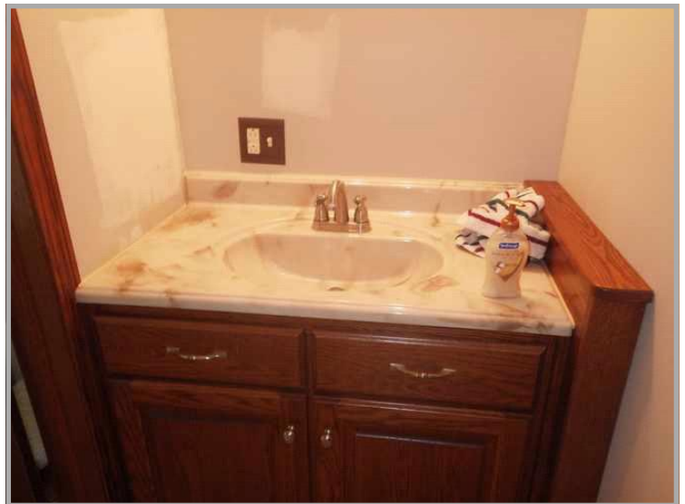
Full Bathroom - Mostly Complete
