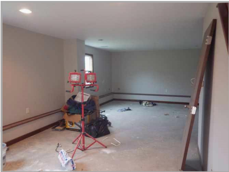
Rec Room - Incomplete Lighting - No Floor Cover
