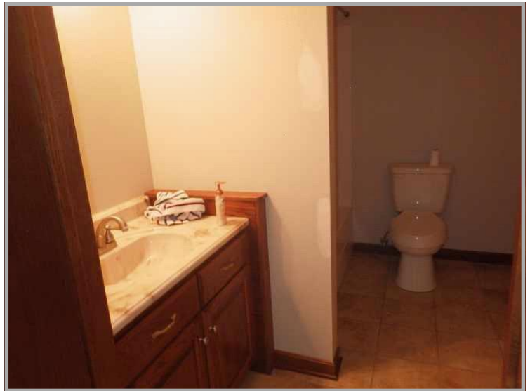
Full Bathroom - Mostly Complete
