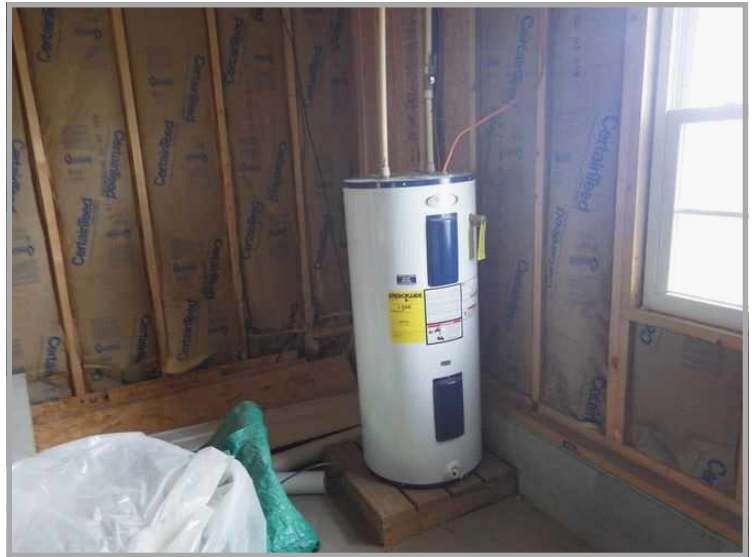
Hot Water Heater in Garage
