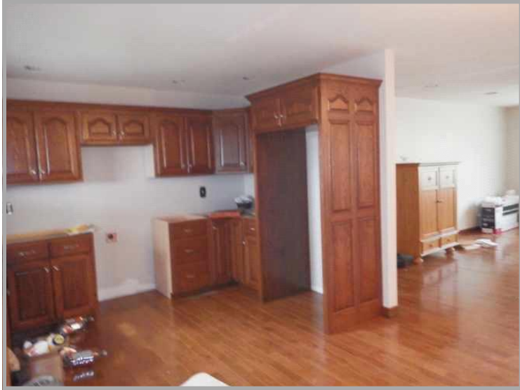
Kitchen - Missing Countertops, Built in Appliances & Incomplete Wiring
