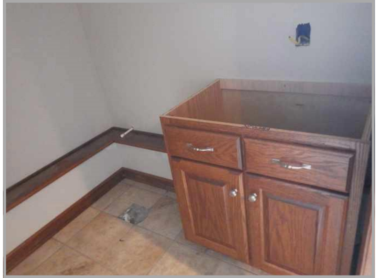
First-Floor Half Bathroom - Incomplete Wiring - No Toilet or Sink Top
