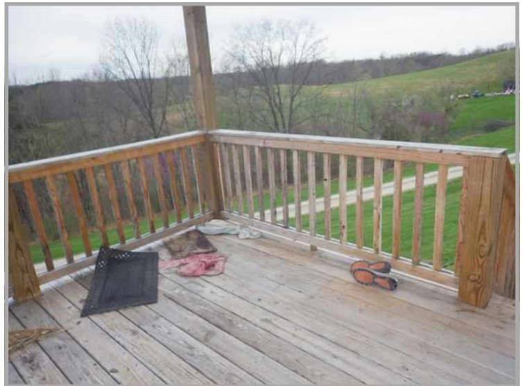
Covered Wood Porch
