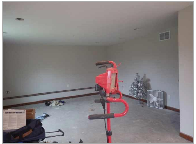
Rec Room - Incomplete Lighting - No Floor Cover
