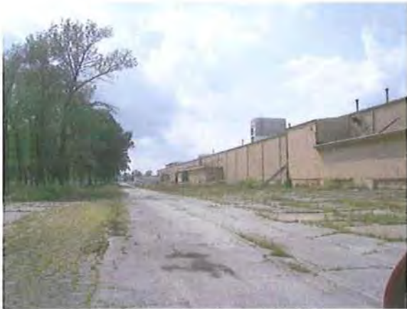
South Side of Uniroyal Building
