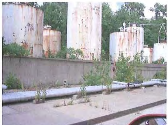
Secondary Containment Around AST - Farm
