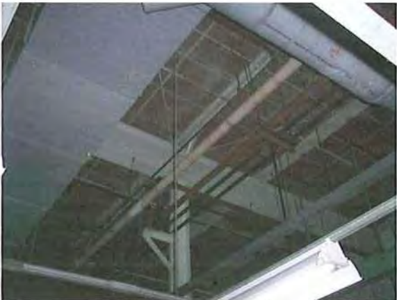
Ceilings in Office Area
