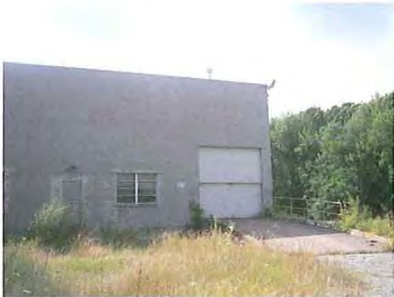
East end of Main building
