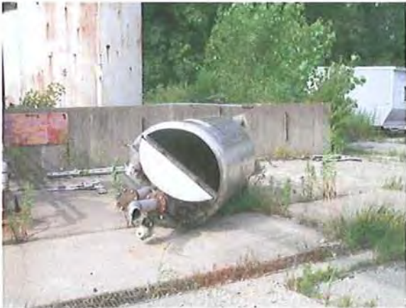
Secondary Containment Around AST Tank Farm
