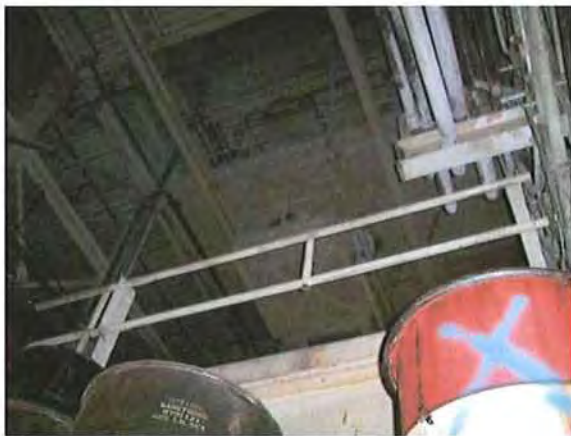
Suspect Asbestos Piping
