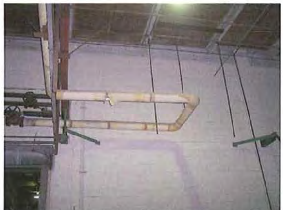
Suspect Asbestos Piping
