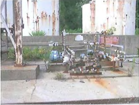
Above Ground Tank Piping
