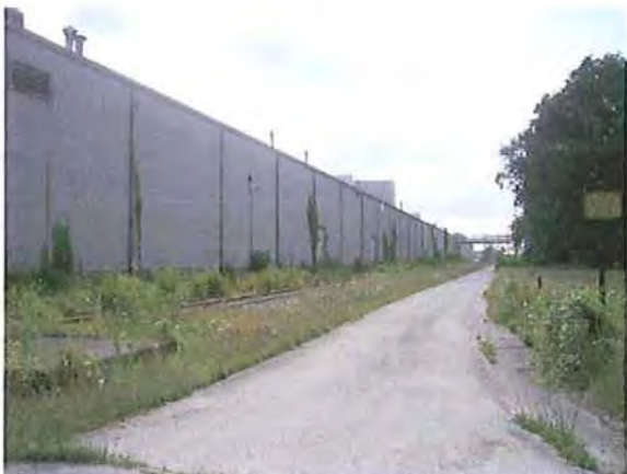
North side of Main Building
