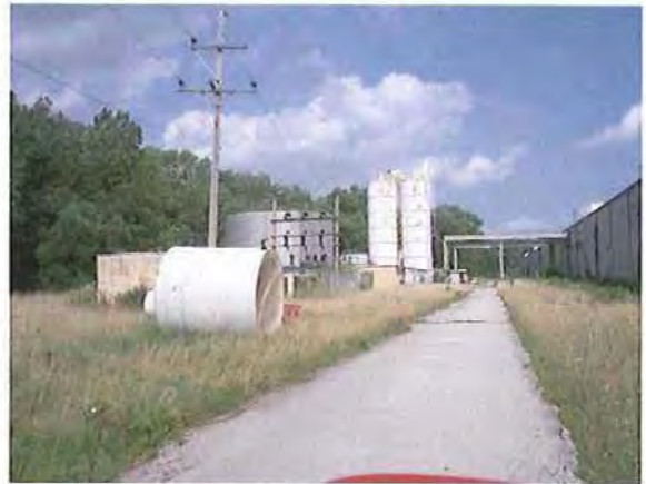
Above Ground Storage Tank Area
