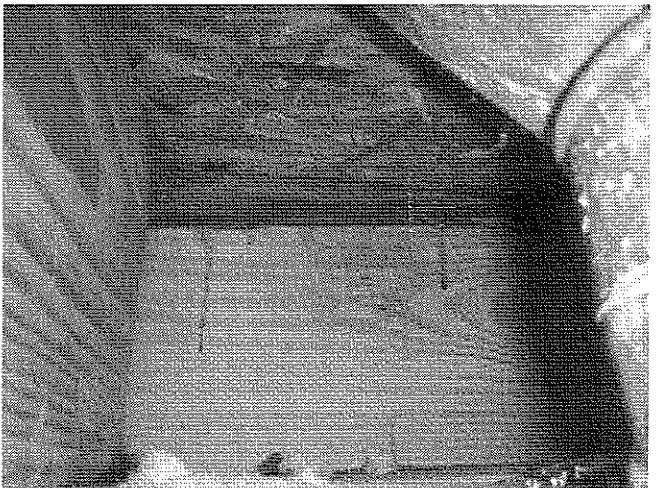
Item 10. Moisture staining on band joist under den/office window.
