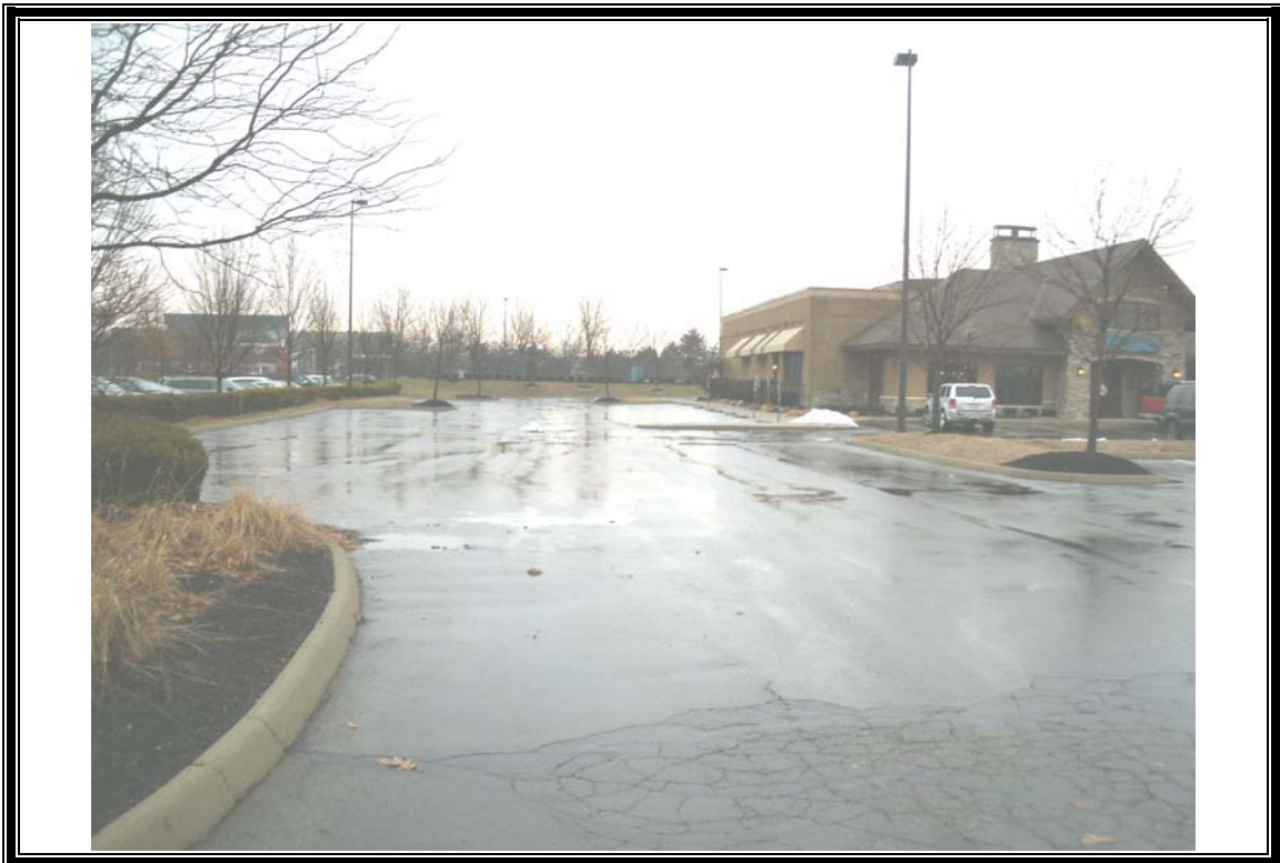
Photo 6: March 10, 2010 Viewing north across the western side of the property.
