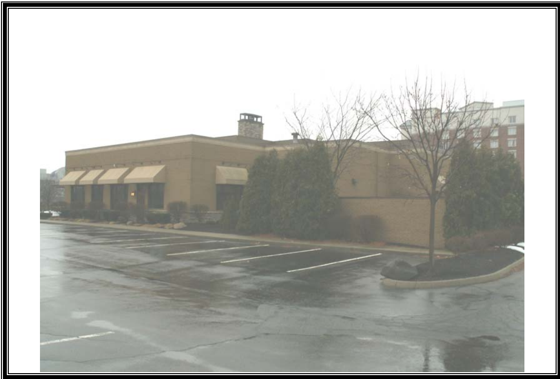
Photo 3: March 10, 2010 Viewing southwest at the eastern side of the restaurant building.
