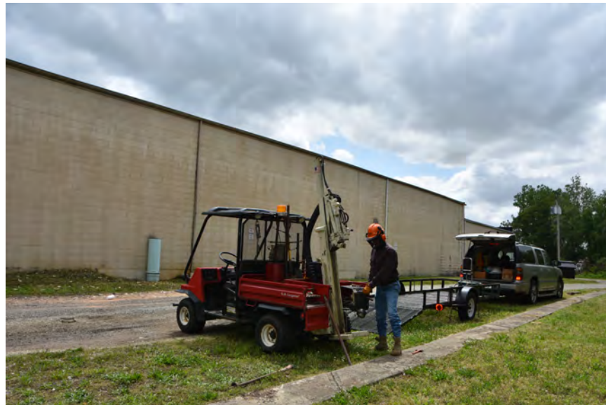
Installing boring GP-1.
