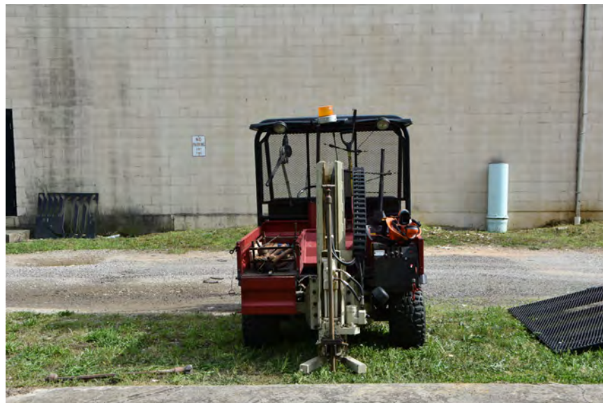
Installing temporary well GP-1
