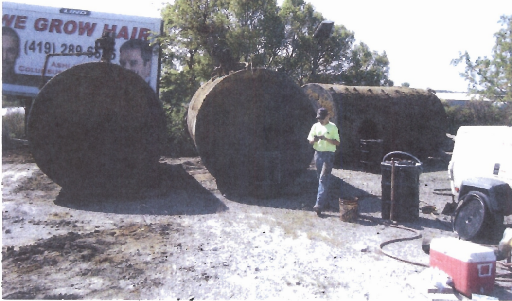
PHOTOGRAPH 1. View of the gasoline USTs #1, #2, and #3 following removal.
