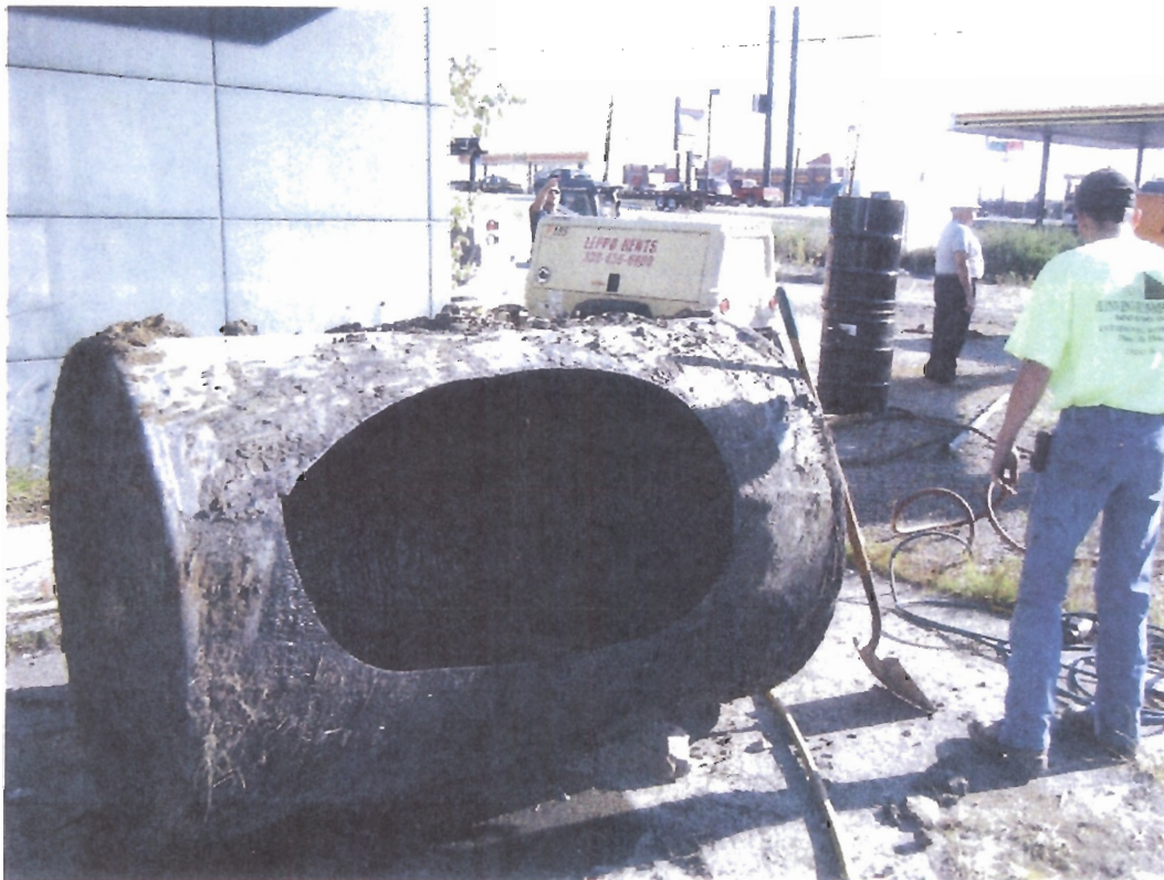
PHOTOGRAPH 2. View of UST #4 following removal.
