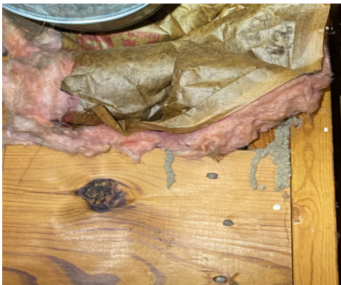
Termite Damage
