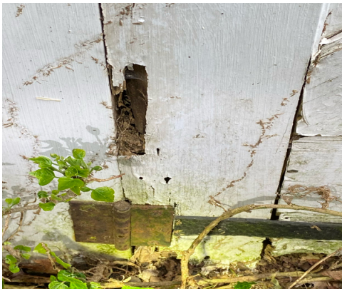
Termite Damage
