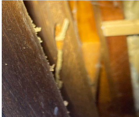
Termite Damage
