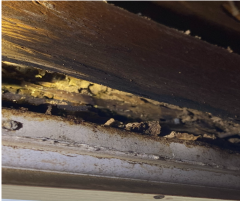
Termite Damage
