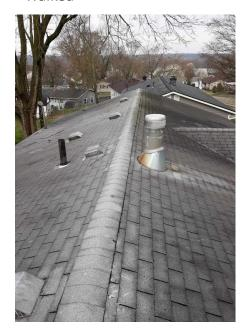
**Roof: Material** 3-Tab(18-22Yr.), Asphalt-Fiberglass **Roof: Material Age** 15-20Yr.
