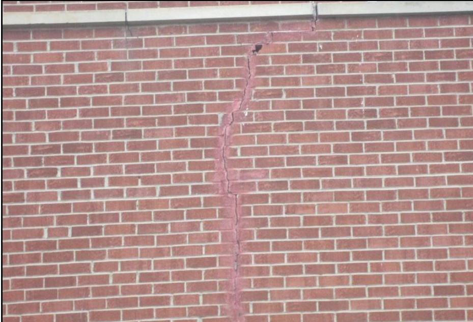
CRACK IN BRICK
