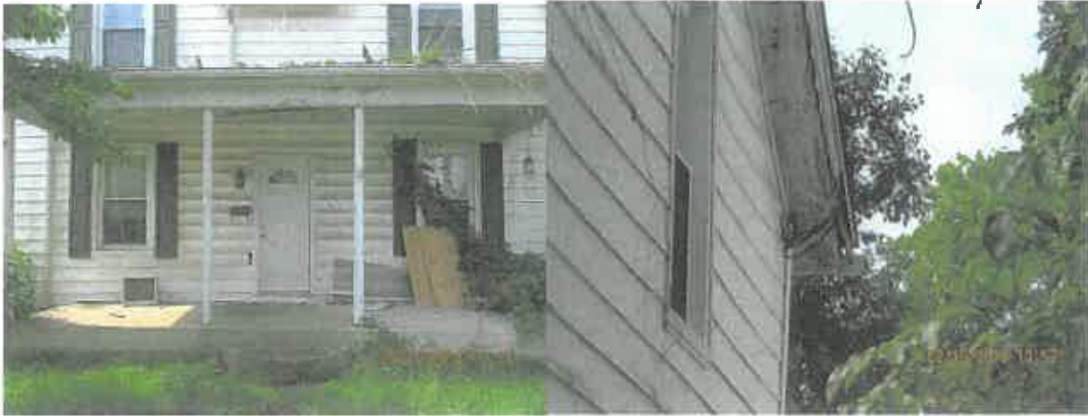
Front porch area last summer
