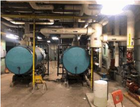
Subject Basement –Hot Water Boiler
