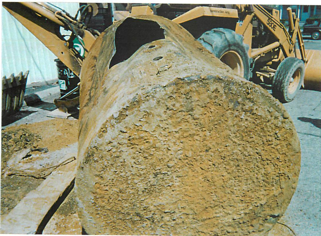
Former 550-gallon used oil UST. Note UST was in good condition when removed from ground.
