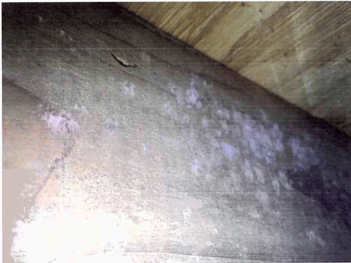
Improper bath vent terminus in attic.
