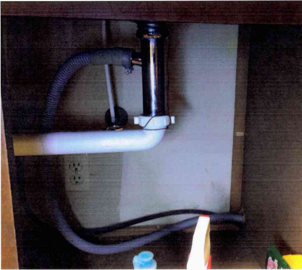
Lack of high loop in dishwasher drain hose.
