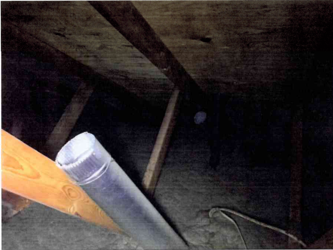
Improper bath vent terminus in attic.
