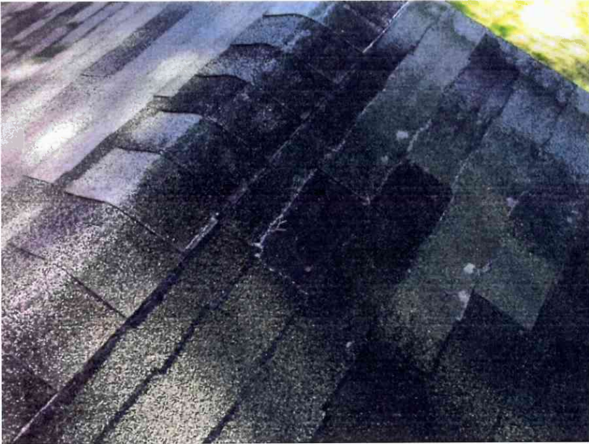
Missing/torn shingle
