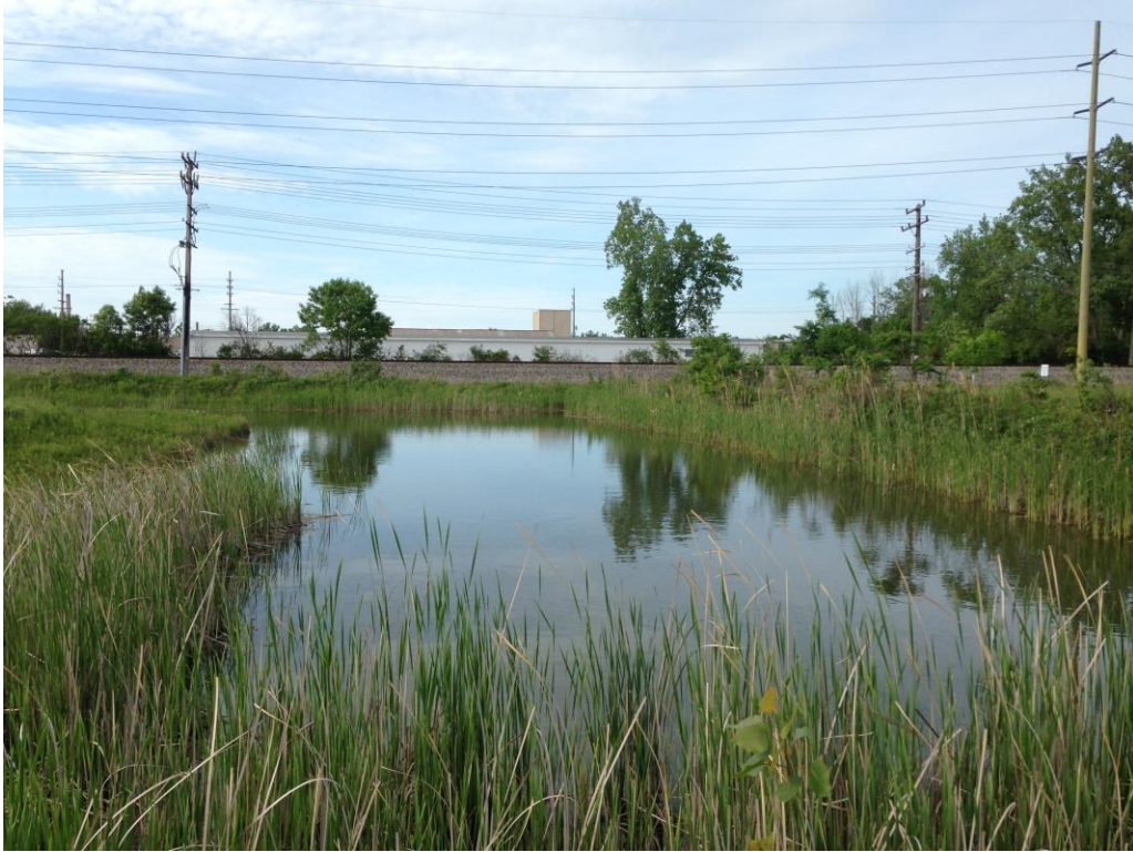
Photo 9. Storm water retention basin within the project area.
